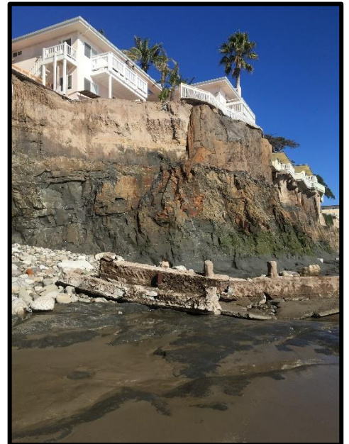
Unpermitted development and construction debris on the beach
