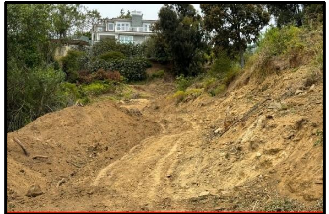
Unpermitted grading and development in ESHA
