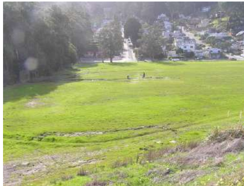
January 19, 2006. Manual excavation of drainage ditches in flooded field at the east end of the field. Grass grows above water surface. Water in bare spots can be seen as reflected sunlight on the field; emergent unvegetated mud is dark brown.
