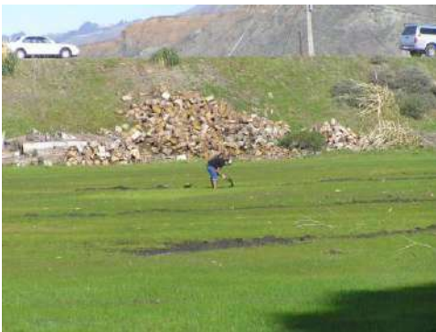
January 19, 2006. Manual excavation of drainage ditches in flooded field at the east end of the field. Grass grows above water surface. Water in bare spots can be seen as reflected sunlight on the field; emergent unvegetated mud is dark brown.
