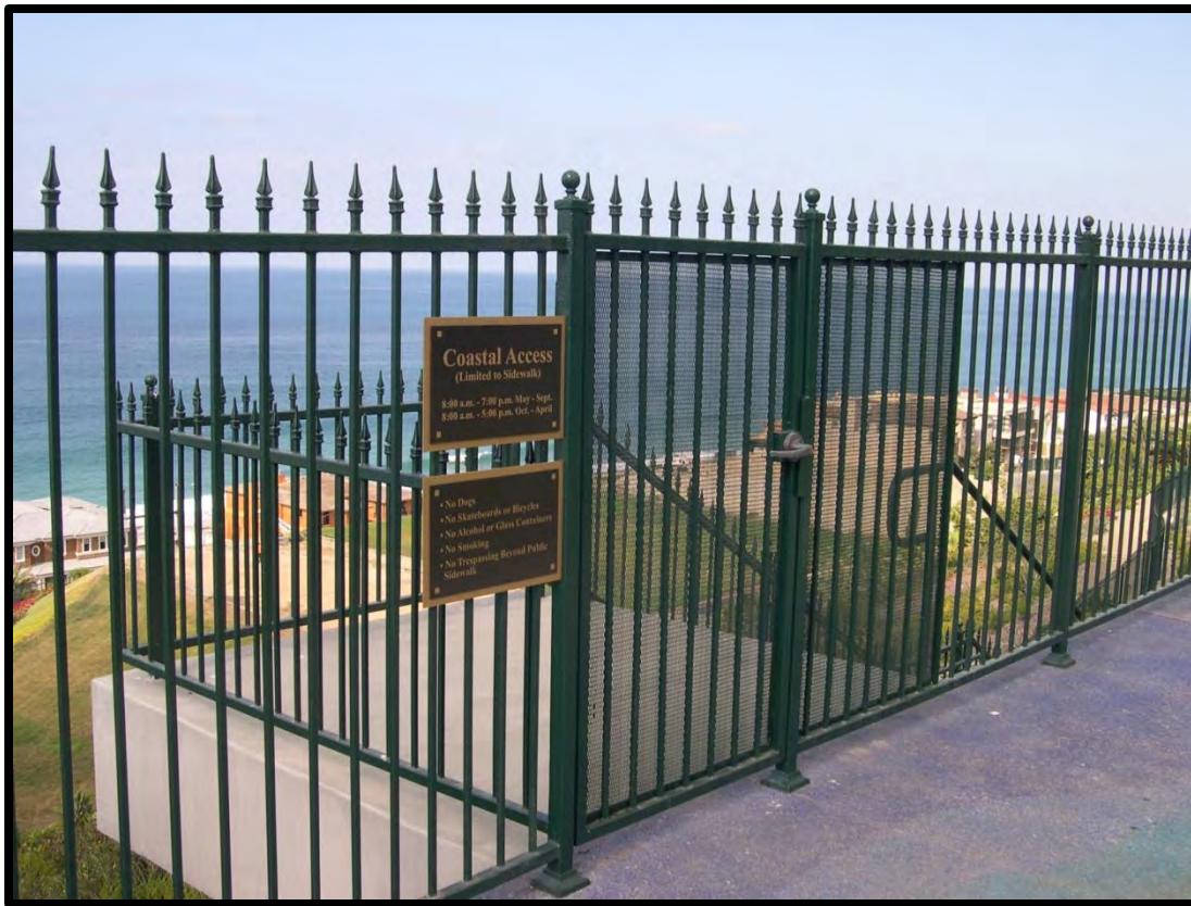
Unpermitted Gate at Mid Strand Beach Access
