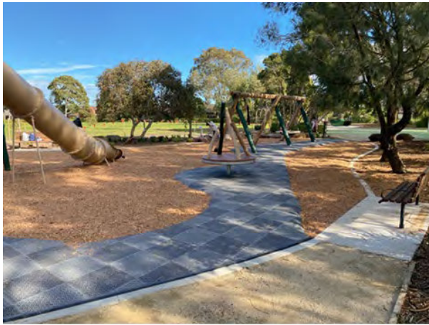
Left: Interlocking PVC tiles integrated with loose-fill playground surfacing for wheelchair accessibility and as scuff pads below playground equipment. 72 Right: Interlocking PVC tiles used for playground surfacing at a Los Angeles public school. 73
