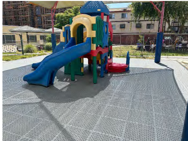
Left: Interlocking PVC tiles integrated with loose-fill playground surfacing for wheelchair accessibility and as scuff pads below playground equipment. 72 Right: Interlocking PVC tiles used for playground surfacing at a Los Angeles public school. 73
