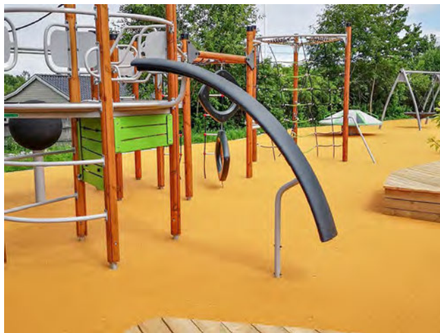
Left: Engineered Wood Fiber playground surfacing. 67 Right: Poured-in-Place cork playground surfacing. 68
