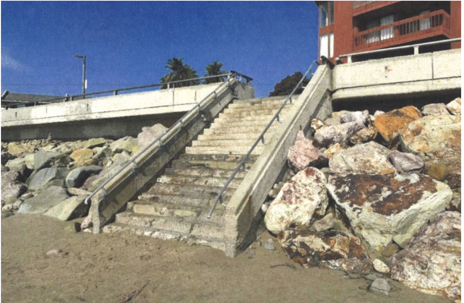
Existing Staircase Photo 11.1.2022
