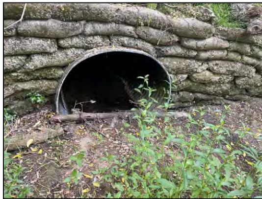
Figure 1 – Photo of the 48" existing pipe and headwall, taken February 2024
