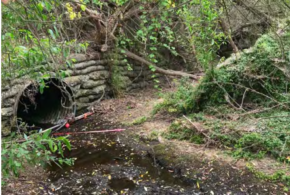
Exhibit 6. Photograph dated 5/31/2018, taken by Anita M. Hayworth of DUDEK, showing the headwall and upper end of 48-inch corrugated metal pipe at the upper end of the former blue-line stream.
