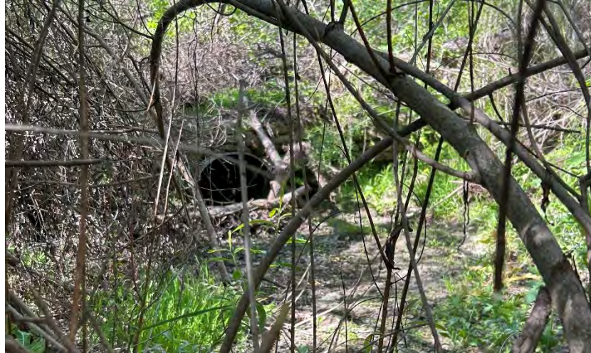
Figure 3: The headwall and 48" pipe at the northeast end of the subject site, taken from the property north of the subject site looking south towards the subject site.
