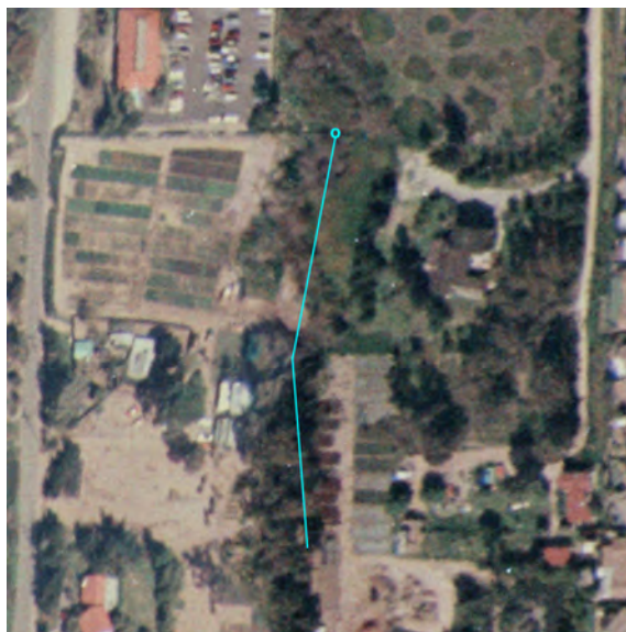
Exhibit 4. 1984 aerial image with the approximate locations of the headwall and the northern half of the 48-inch CMP alignment indicated in cyan. At that time, the upper reach of the future pipe alignment passed through an s-shaped streambed.
