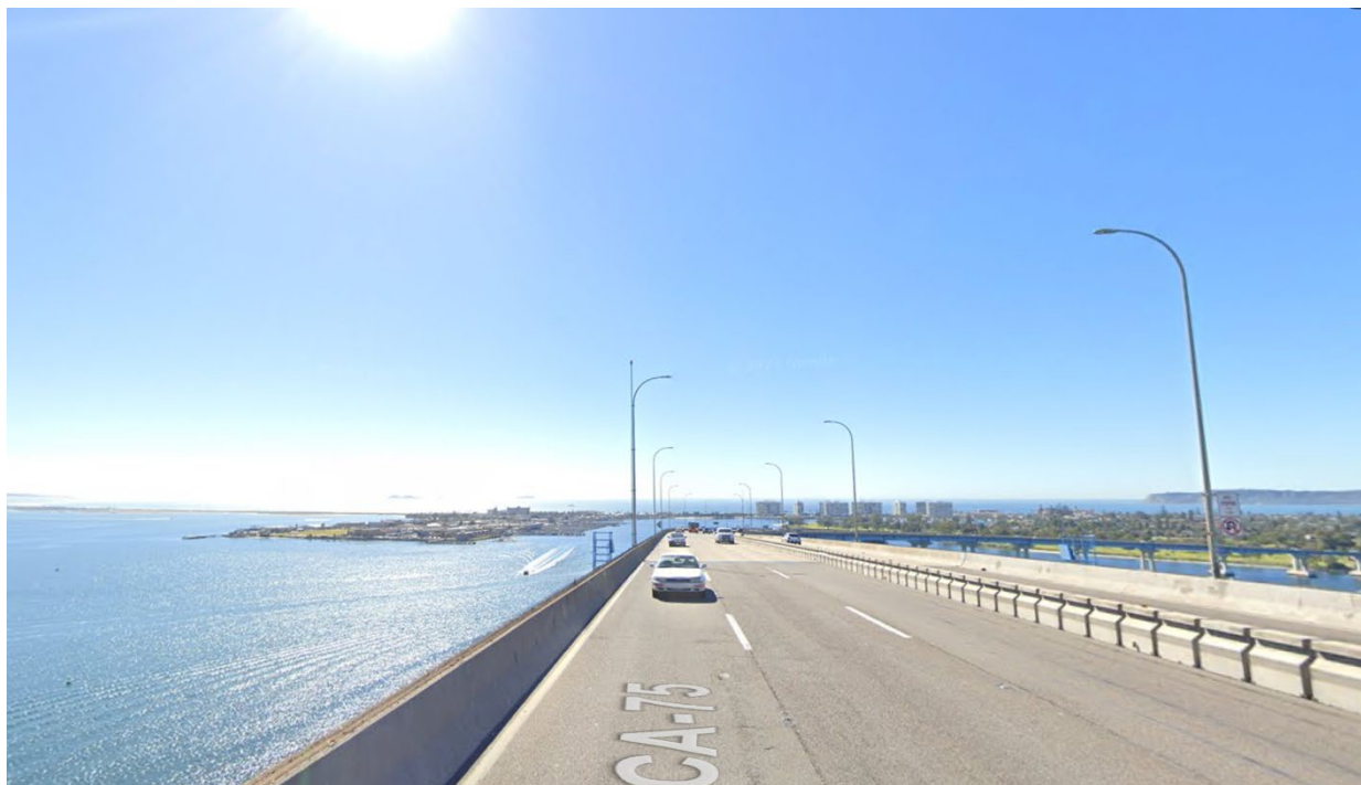
Figure 1: Existing Bridge Conditions
