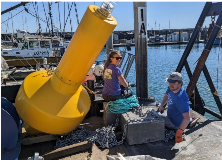
Figure 2 PATON marker buoy and the pair of concrete clump weights prior to deployment.
