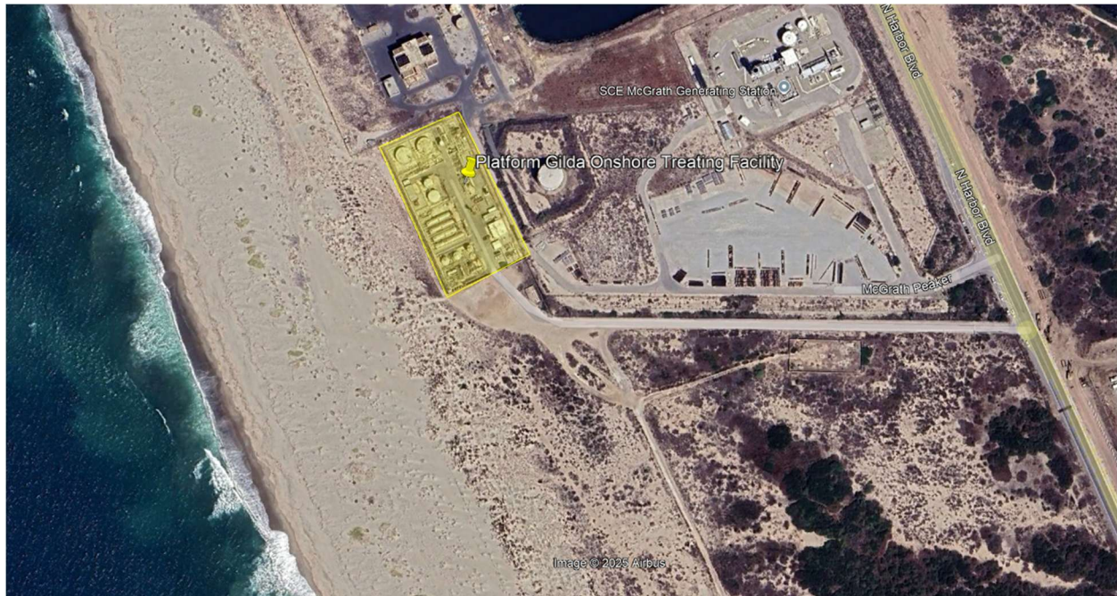
Figure 10. Existing Onshore Treating Facility located in sensitive dune habitat. 440
